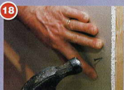
18 Make sure the nails are knocked well in and flush with the surface; take care not to make dents around the nail – what used to be called 'half-crowns'
